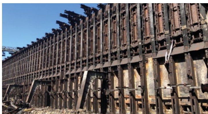
Batteries undergoing demolition
