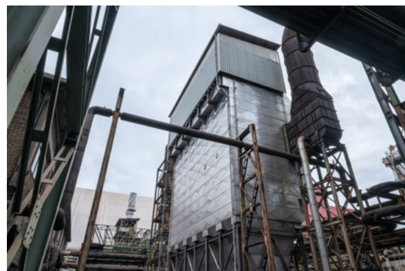
New fume dedusting installation on stack E424
