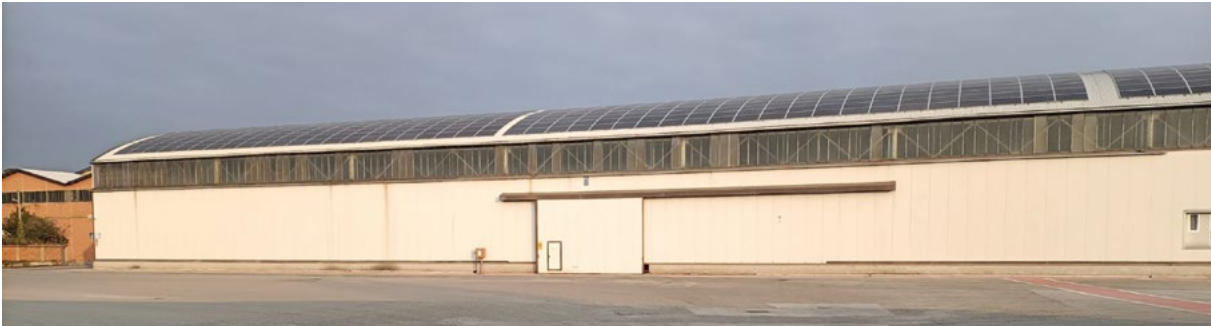
Plant building and photovoltaic system of 596 kW on the roof
