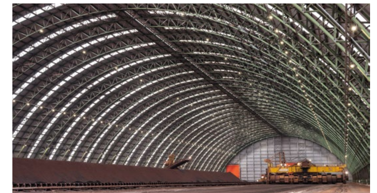
Enclosure of ore blend stockyard
